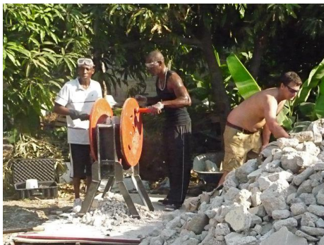
Crushing rubble into usable aggregate
