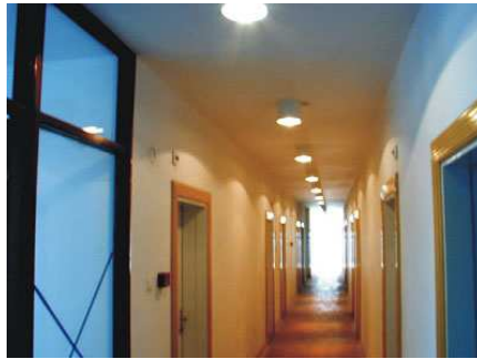
Figure 8: Typical category B luminaire when intended for use in office corridors (outside the product boundary).
