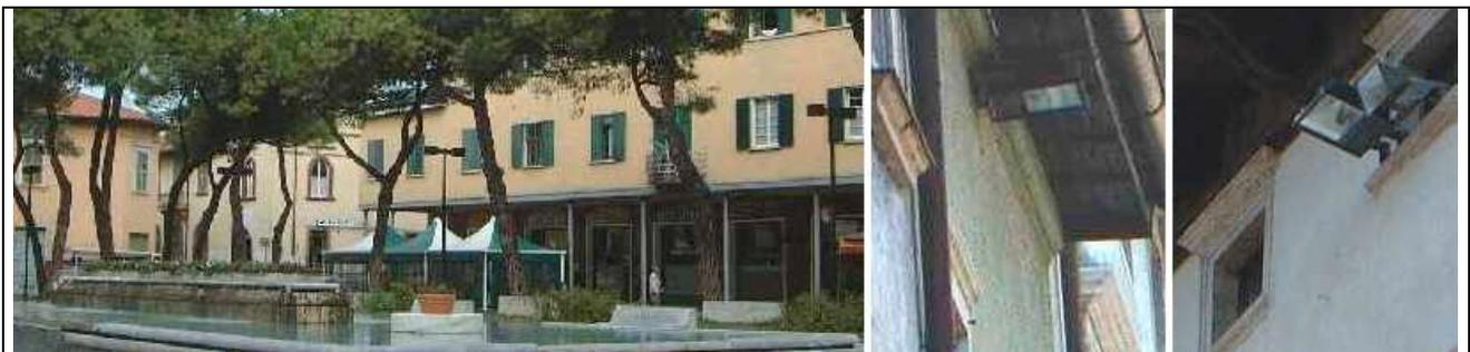
*Fig.11 – Left: Dalmine City Hall Square. Lighting corresponding to the R.L. 17/00 requirements and light sources placed so as not to interfere with the trees canopy. Right: Two examples of lighting of old cities centres with devices under eave (in the image to far right a horizontal device put beside to an inclined one which instead disperses light upwards).*
