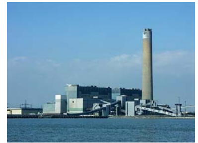
Figure 23.1. Coal being delivered to Kingsnorth power station (capacity 1940 MW) in 2005. Photos by Ian Boyle www.simplonpc.co.uk .
