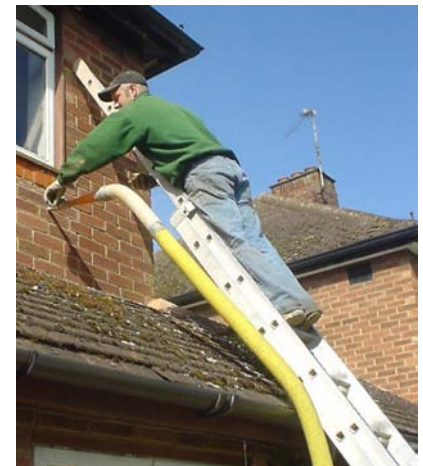
Figure 21.5. Cavity-wall insulation going in.
