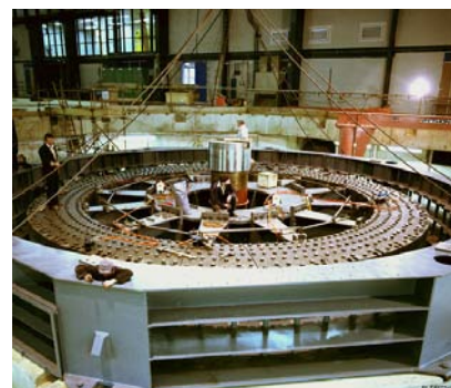
Figure 26.15. One of the two flywheels at the fusion research facility in Culham, under construction. Photo: EFDA-JET. www.jet.efda.org .
