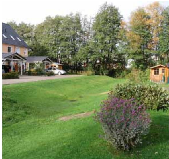
Muldenversickerung in Brokhuchting.
