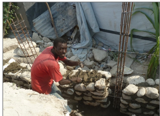
BWB's Rodney Constant lays the stone base of the site wall.
