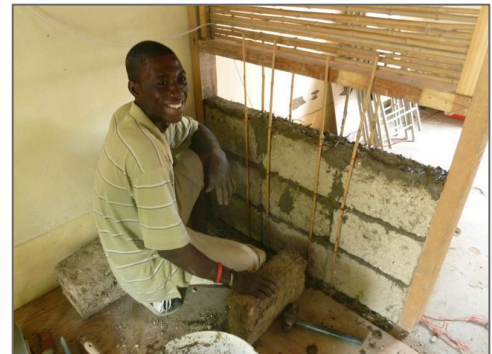
BWB's Jean Louis Elie installs a new earth-block and bamboo partition in the Ti Kay Pay.
