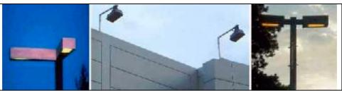
*Fig.14 - The figures show some devices for road , car parks and industrial sheds lighting. The lamps used are full cut-off, low-pressure sodium equipped with horizontal flat glass.*
